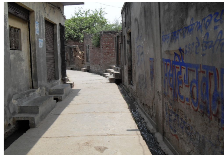
OPEN DRAINS ON BOTH SIDE OF STREET
