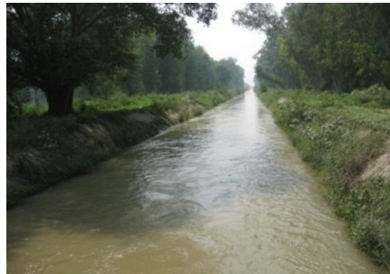
Fig No. 45:- Downstream of Sabhraon Branch
