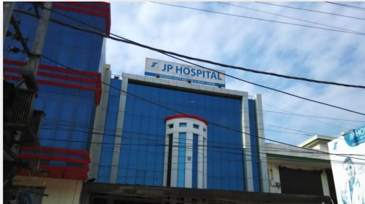
Figure 9 Multispecialty JP Hospital in Zirakpur
